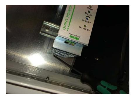
• Reinstall middle plate. Remember the earth connections under one of the bolts.
